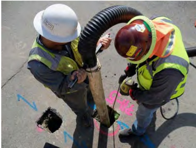
C Below technicians performing potholing
